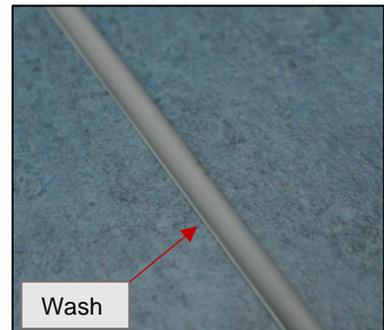
**11.1.8.** Using a trim plate, make the first pass while the welding rod is still warm. If the rod cools down too much the force of pushing the knife through it can cause it to pop out.
